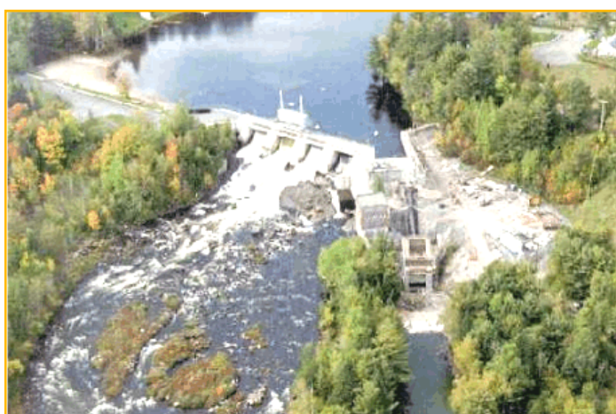
Figure 8: Mini Hydro with high head; Photo credit: SNC lawalin: www.retscreen.net
